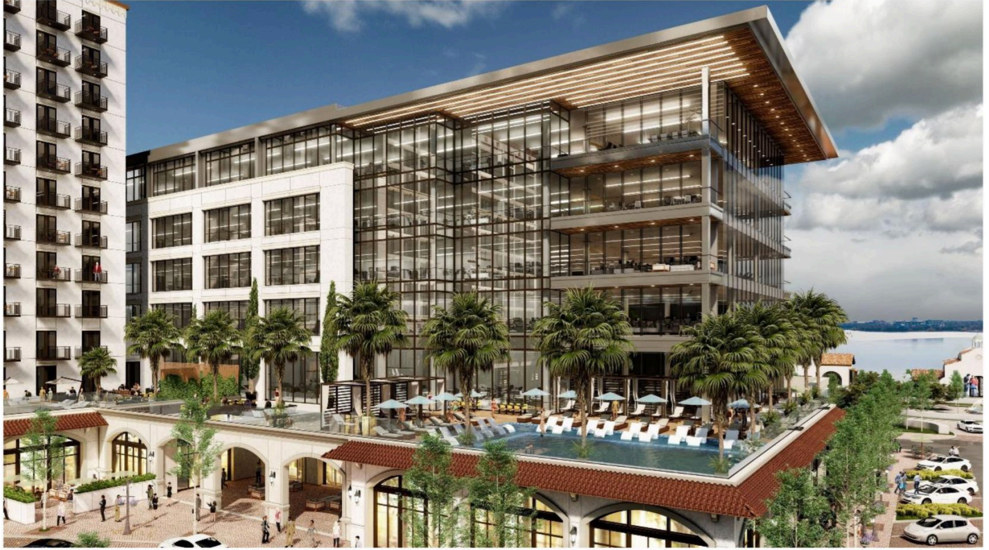
The six-story office building will include a private club. (Merriman Anderson Architects )
